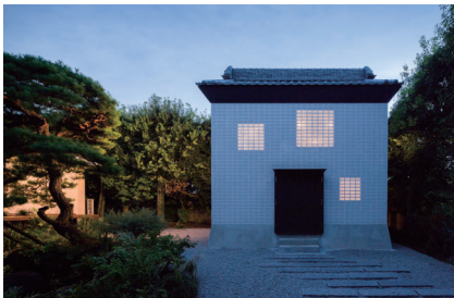
Title : Rebirth House Location : Moriya-shi, Ibaraki Usage : Assembly salon Total floor area : 41m 2 Structure : RC Completion : 2014
