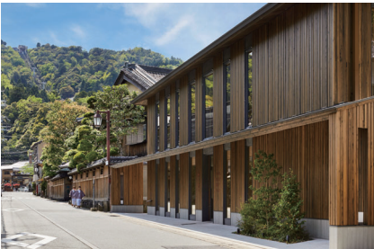
Title : SANPOU Nishimuraya Location : Kinosaki, Toyooka-shi, Hyogo Usage : Salon, Restaurant, Shop Total floor area : 468㎡ Structure : Wood Completion : 2019
