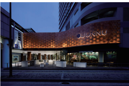
Title : CHIBA SOGO | JUNNU Location : Chiba-shi, Chiba Usage : Department Store Total floor area : 10,279㎡ Structure : RC Completion : 2017
