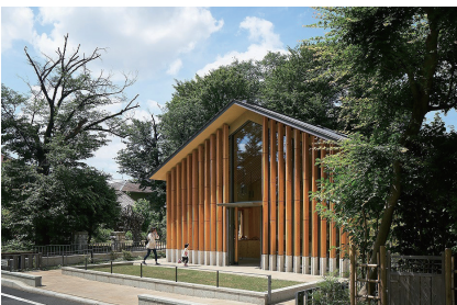
Title : JIYU GAKUEN MIRAIKAN Location : Higashikurume-shi, Tokyo Usage : Education Total floor area : 353㎡ Structure : Wood Completion : 2017
